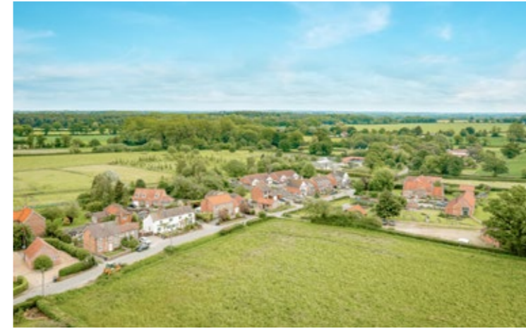
Aerial view of The Old Chequers and surrounding area
