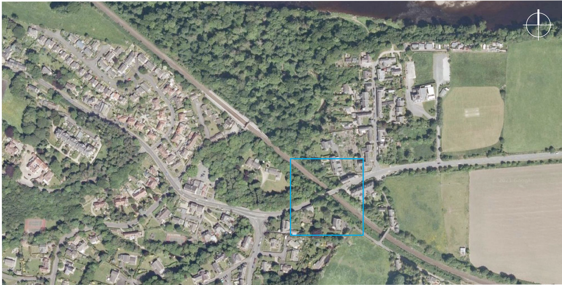
Fig 2 Aerial view of development site
